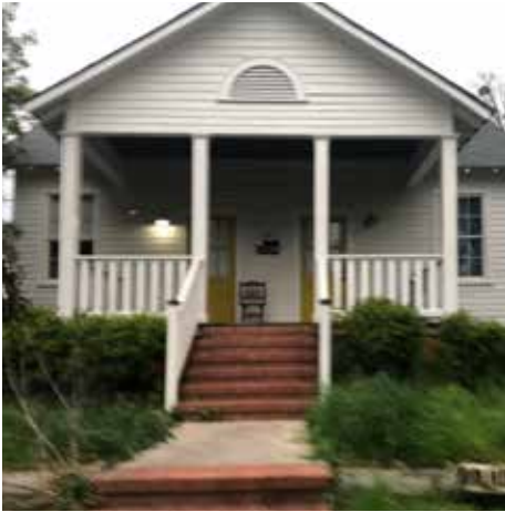
Renovated housing for artists in the Mill Hill neighborhood of Macon.
