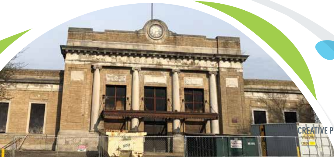
Train station under redevelopment in Wilkinsburg.
