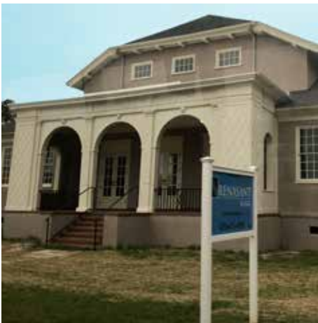
The Mill Hill Community Arts Center in the East Macon Arts Village AFTER its renovation.
